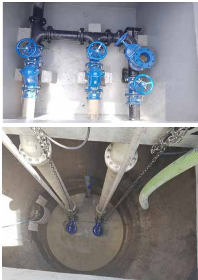
Work is in progress at sewage pumping stations
